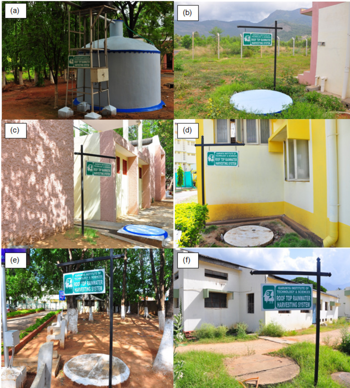
Figure 3. Soak pits located at (a) Administrative block (b) Aero space lab (c) Civil lab (d) Guest house (e) Hepzibah hostel and (f) Father Duraisamy Residence hostel
