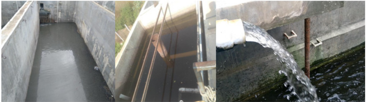
Figure 13 JMR collection tank, settling tank (after filtration)
